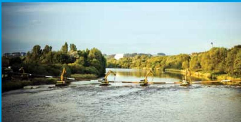
VolkerStevin completing the construction and installation of a 132m long, 609mm diameter pipeline during low tide across the River Lune, Lancaster.
