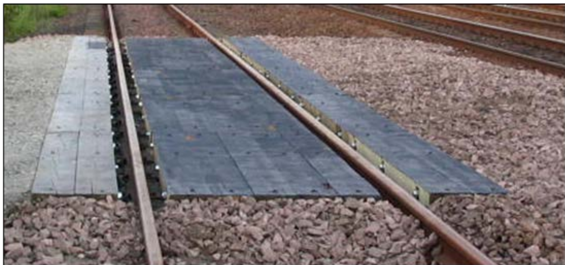
Illustration 5 - Secured timbers level with the rail head
