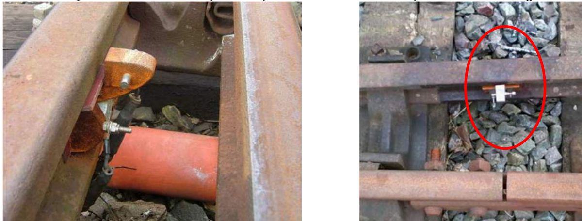
Figure 2. examples of Track Circuit Interrupters
